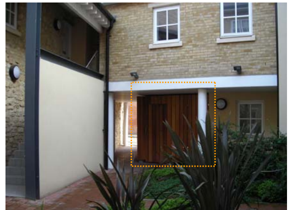
Secure residential cycle storage compound (Bookbinders Court, Oxford)
