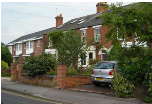
Front garden parking should be integrated into the street scene (Grandpont, Oxford)
